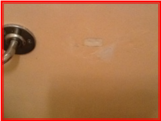
1.4.1 Hole behind door from handle Loose tiles at the bottom of the bath .
